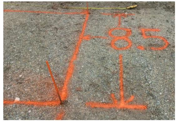
After measuring and placing all four stakes at the corners, lay the grid bundle in the center, around the 12' mark (on 24' long side)
