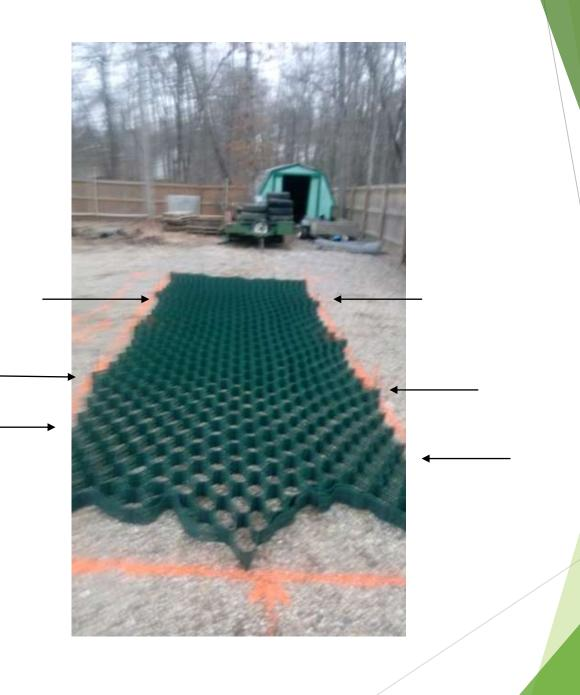
Apply the same technique to the shorter sides. First start in the middle at about the 5th cell (4 - 4.5' to the center)
