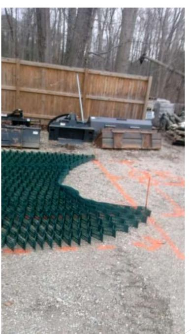
Go to center of grid at 12' (on 24' length side) and stake those cells out at the perimeter.
